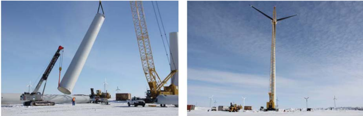
Figure 4. Installation of an EWT 900 wind turbine
